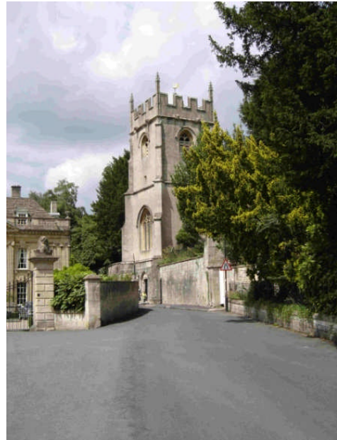
View of the church's tower
